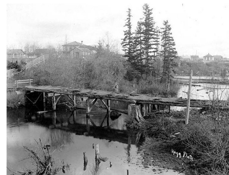
At right: part of the old Military Road, taken by E.A. Hegg, Whatcom County photographer.
